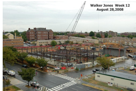
Figure 3 – Steel erection, week 12.
