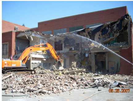
Figure 2 - Demolition of Terrell Junior High.
